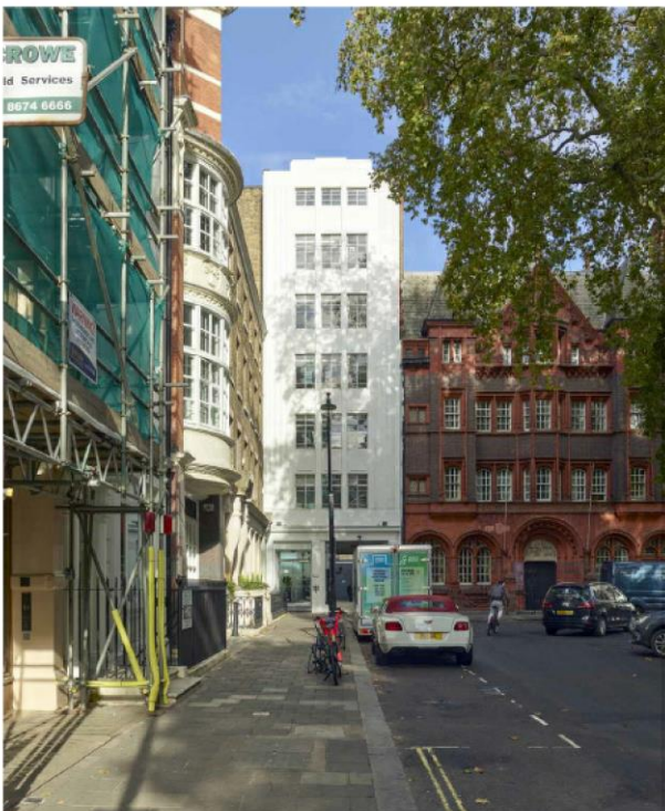
Existing view on Soho Square
